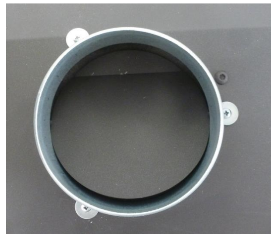
Figure No.8 - Correctly screwed nozzle at the 3 points with the washers
